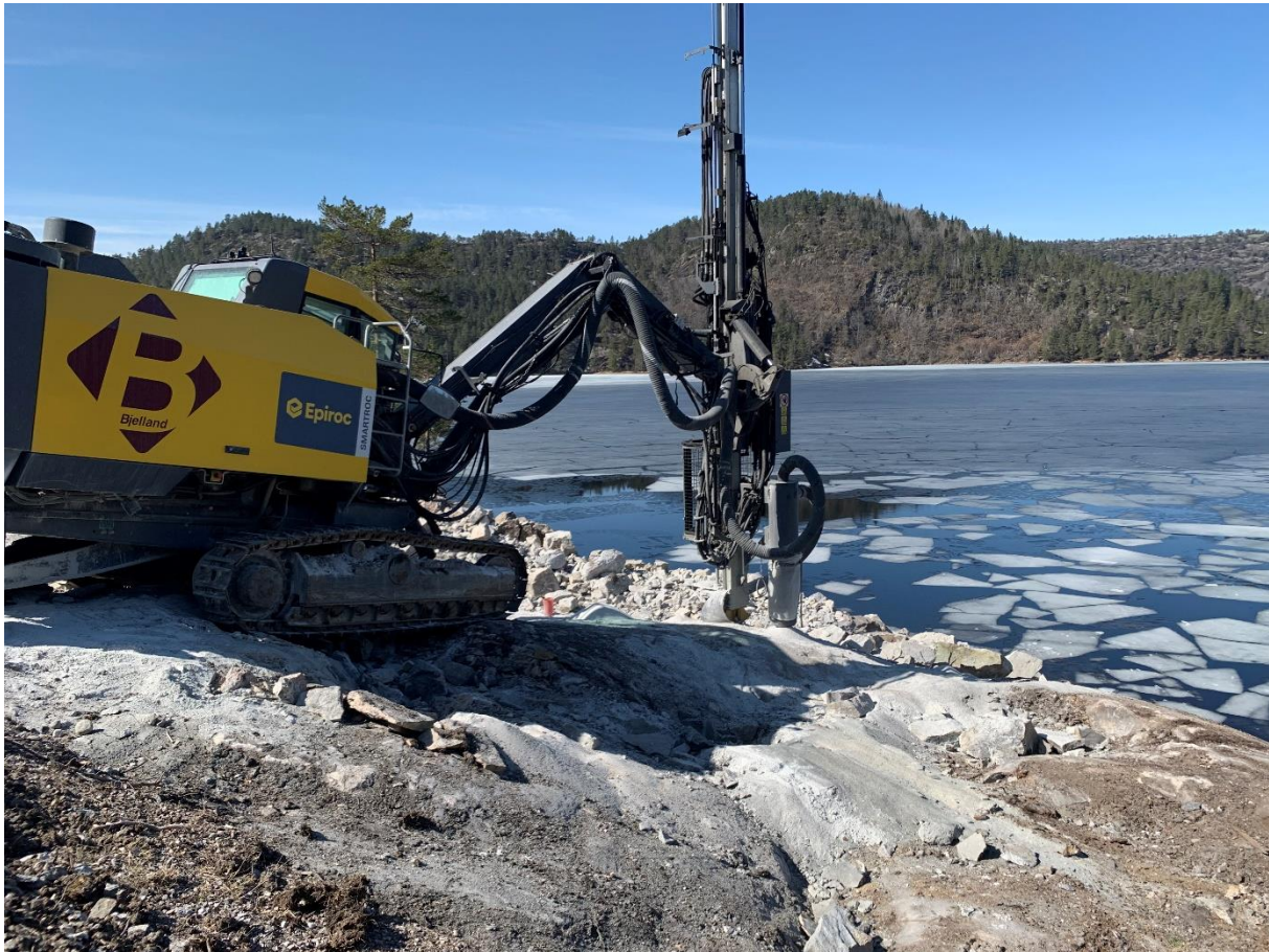
Photo: Eirik Noer Smestad, Flateland Project
