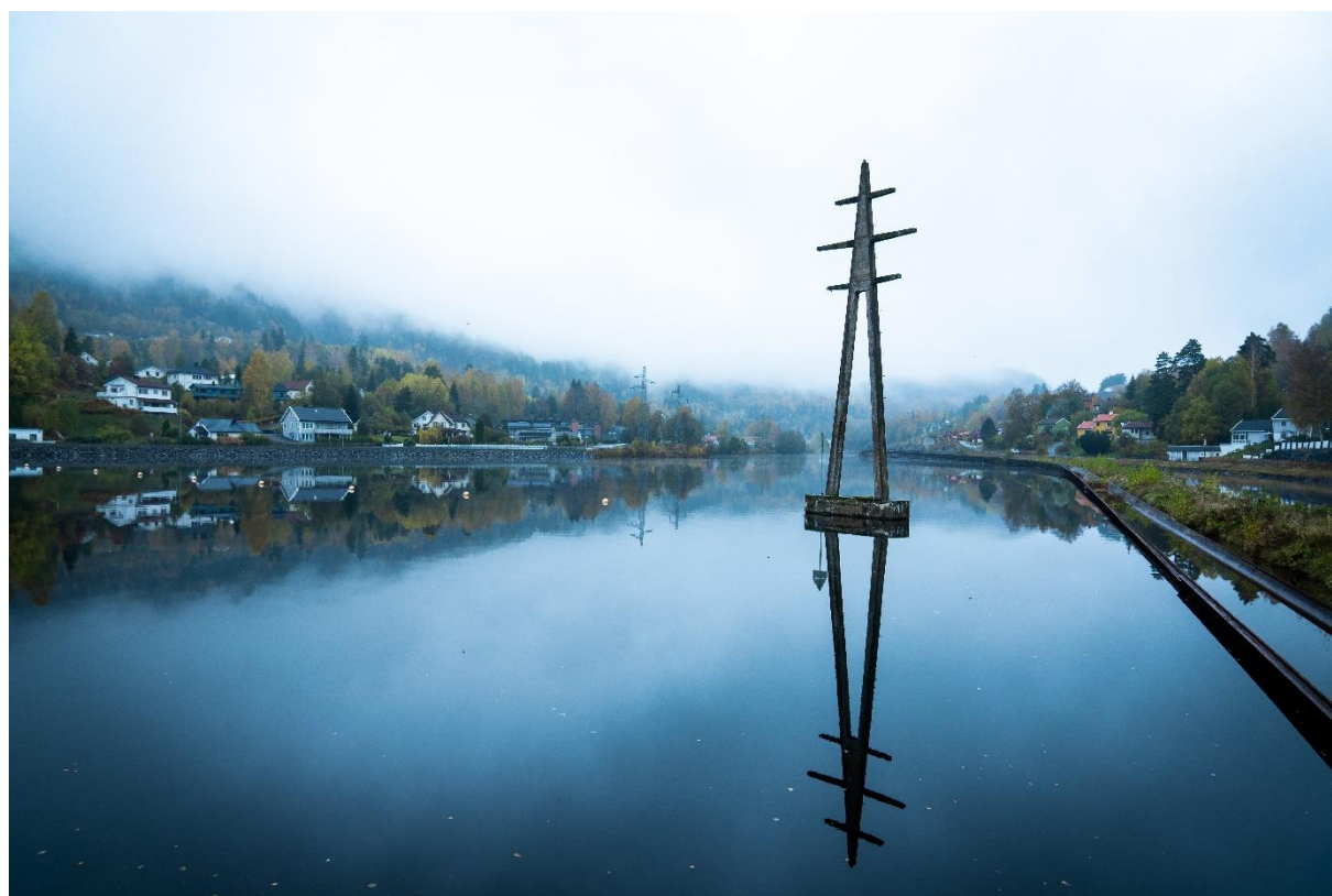
Upstream Tinfos I powerstation, Notodden, Norway
